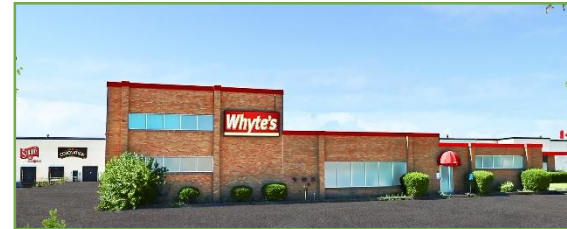
Production and distribution facility (150 000 ft 2 )
