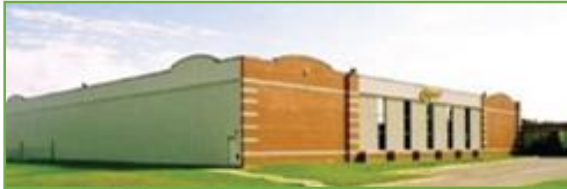
Head office and production facility (60 000 ft 2 )
